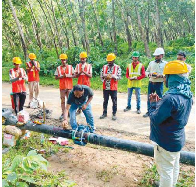
Pipeline laying, GA 11. 56 Tripura
