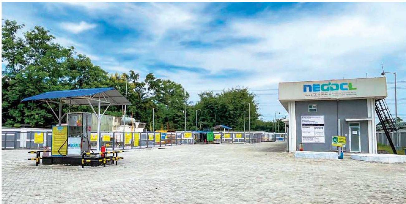
1 st CGS cum Mother Station of NEGDC at Tezpur
