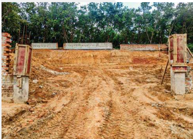
Work-in-progress Anand Nagar CGS, Tripura
